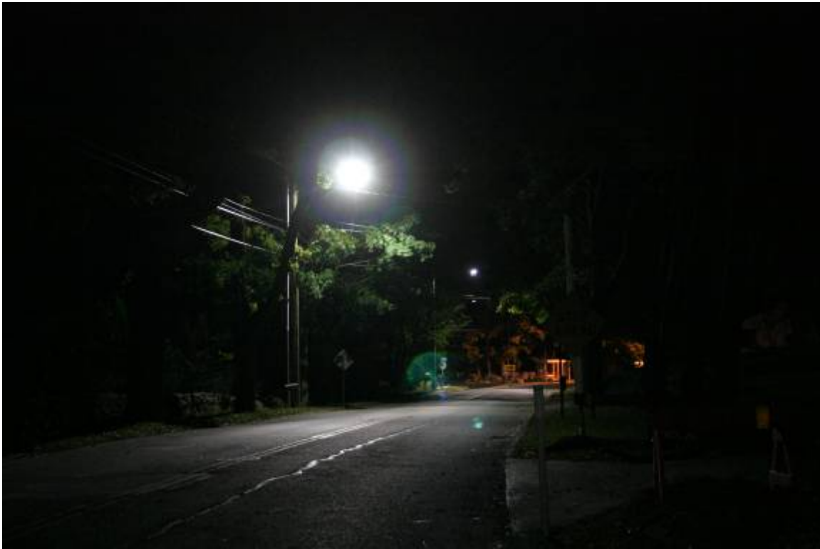
Figure 5. Ceramic metal halide demonstration street lighting (Shennecossett Road)
