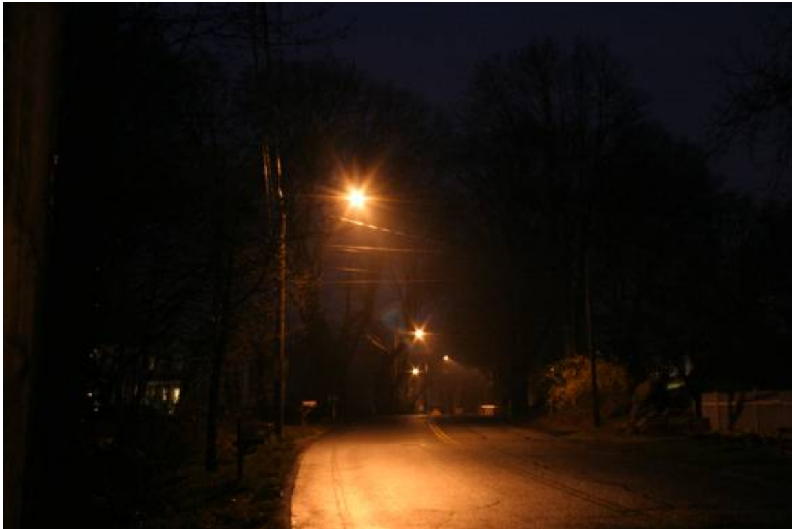
Figure 4. Initial HPS street lighting (Shennecossett Road)
