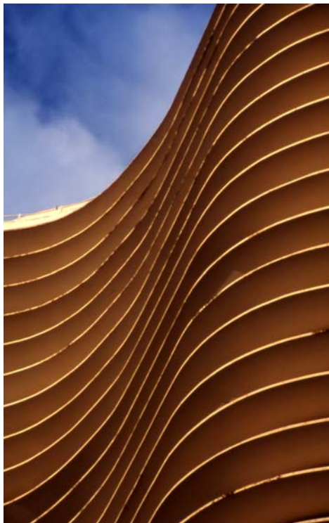
Figure 6. Oscar Niemeyer, Niemeyer Apartment Building (1954-60), Belo Horizonte, brises-soleil .
