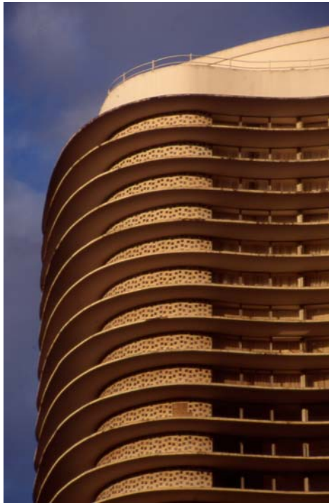
Figure 4. Oscar Niemeyer, Niemeyer Apartment Building (1954-60), Belo Horizonte, brises-soleil and ornamental ceramic tiles.
