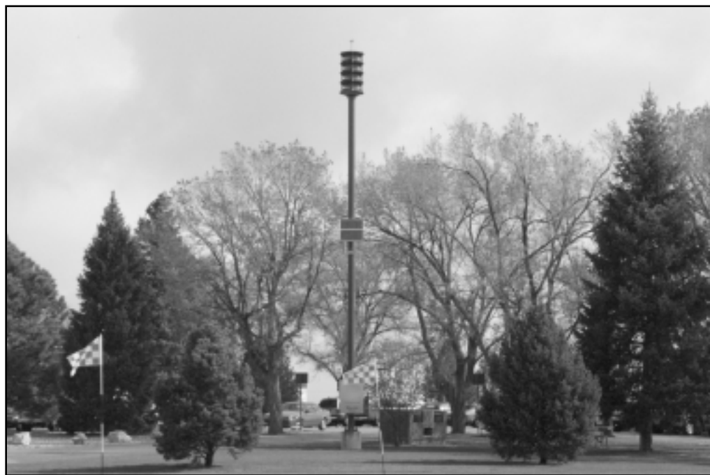
GIANT VOICE towers, like this one on the Silver Spruce Golf Course, will broadcast weekly test sirens at noon each Friday. Announcements for severe weather warnings and Force Protection Changes will also be broadcast via the GIANT VOICE.
