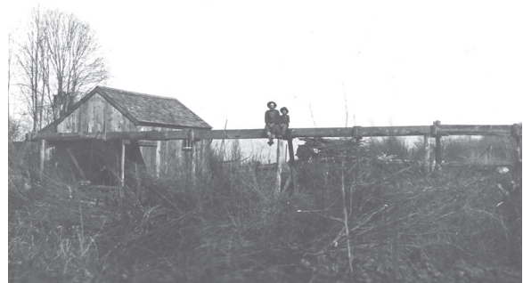
Flume at Bantons' Ladd Canyon ranch, used to provide rotary power to shop tools, such as wood lathe, drill, and sander, 1914 Photo courtesy of Gerald Young
