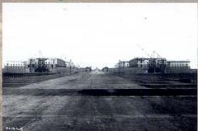
North & South Block under construction.
