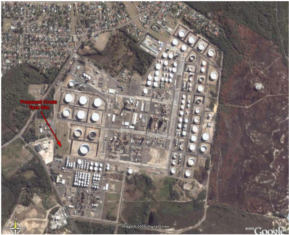
Figure 2 - Aerial View of Proposed Tank Location
