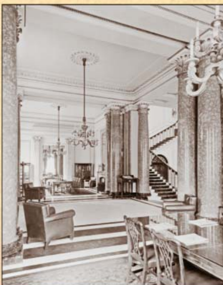
● An early photo of the ground floor foyer
