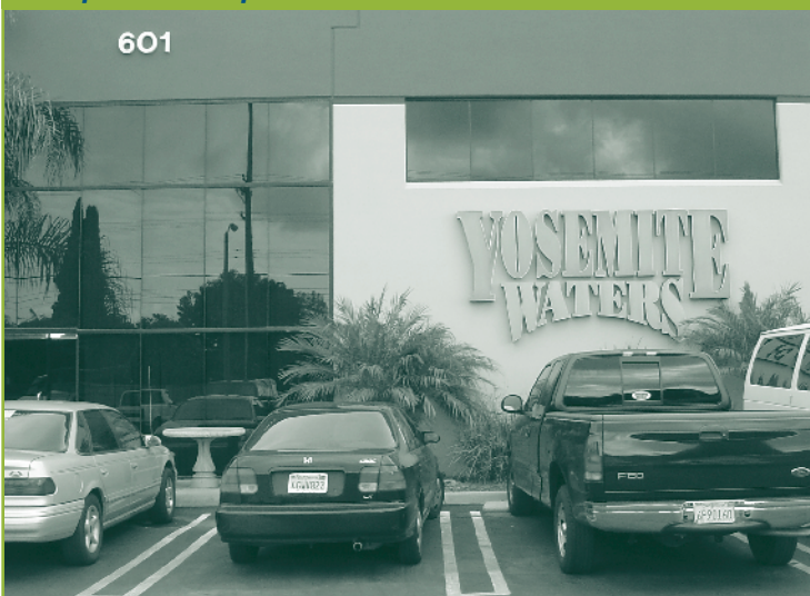
Yosemite Waters' Fullerton Bottling Plant is the company's corporate headquarters.
