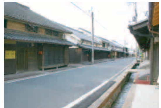
Uda City Matsuyama Preservation District for Groups of Traditional Buildings
