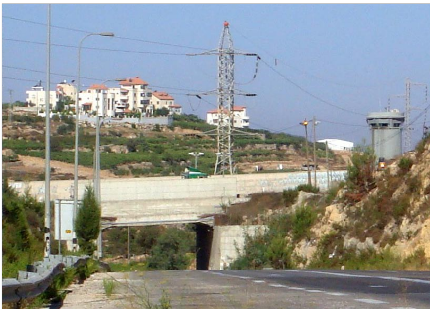
Hallul bridge crosses Road 35 as the map opposite shows. Photo by OCHA, 2007.
