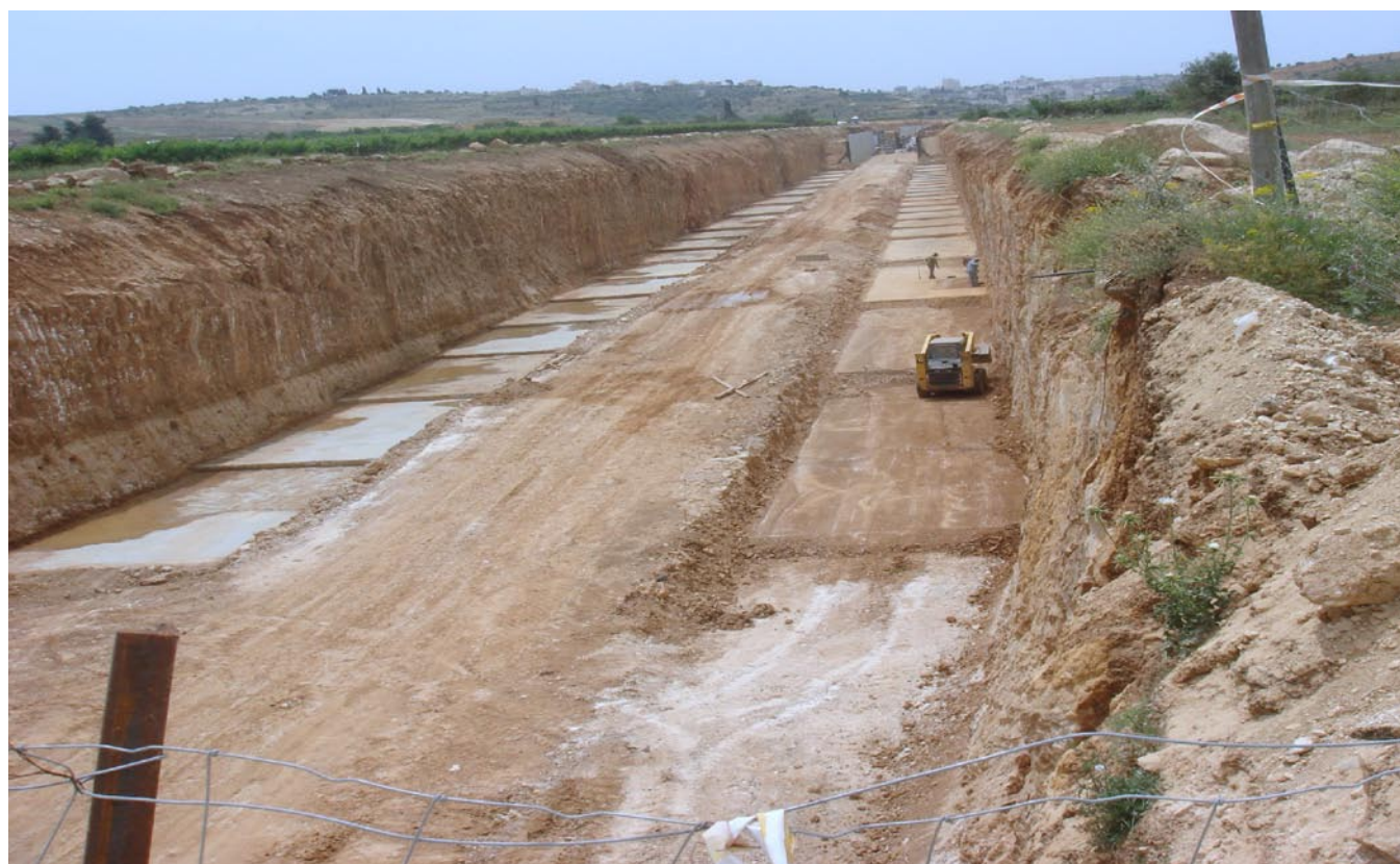
Palestinians wishing to leave the Bir Nabala and Biddu enclaves to travel to Ramallah will need to use a sunken road (under construction) to pass under Road 437, a road reserved for Israeli use. Photo by OCHA, 2007.
