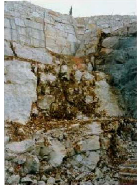
Figure 27. Karstic fractures filled with red-brown soil in the Bina Formation limestone, north portal of tunnels, Begin highway, at the entrance to Jerusalem.
