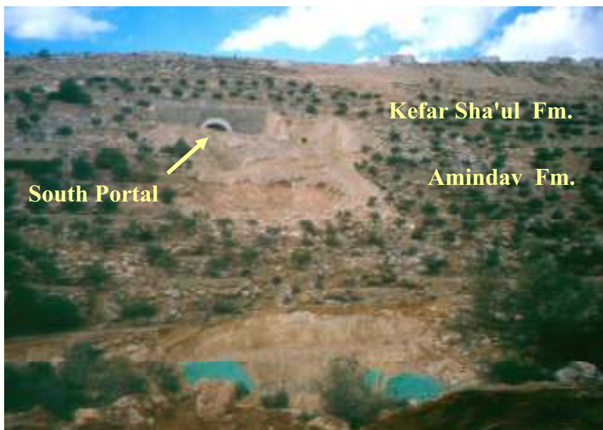
Figure 42. Gilo Short Tunnel south portal in the Amminadav Formation.
