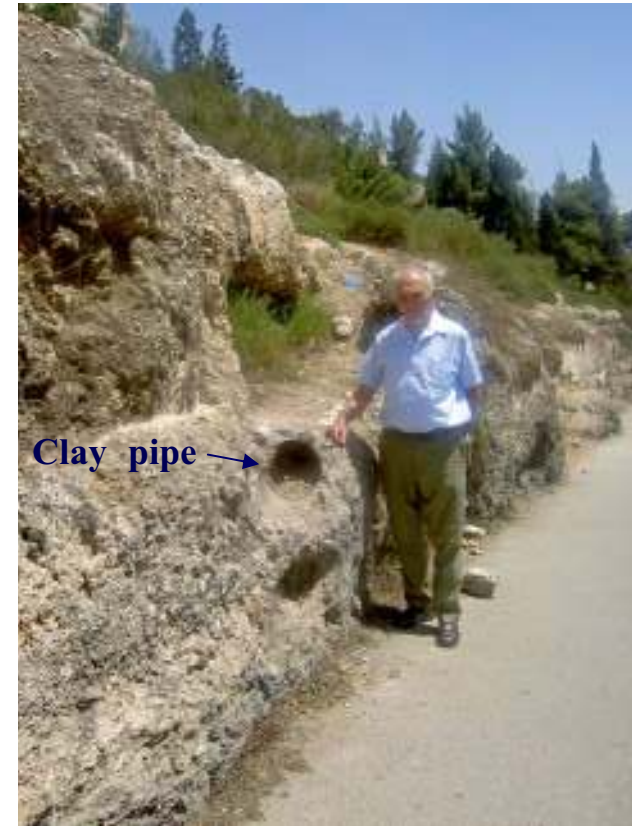
Figure 70. The lower aqueduct between the Sultan's Pool and the Temple Mount located on the western side of Mt. Zion. An Ottoman clay pipe is installed in the aqueduct.
