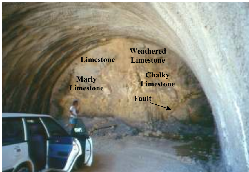
Figure 43. Gilo Short Tunnel work face in the Lower Unit of the Kefar Sha'ul Formation chalky limestone.
