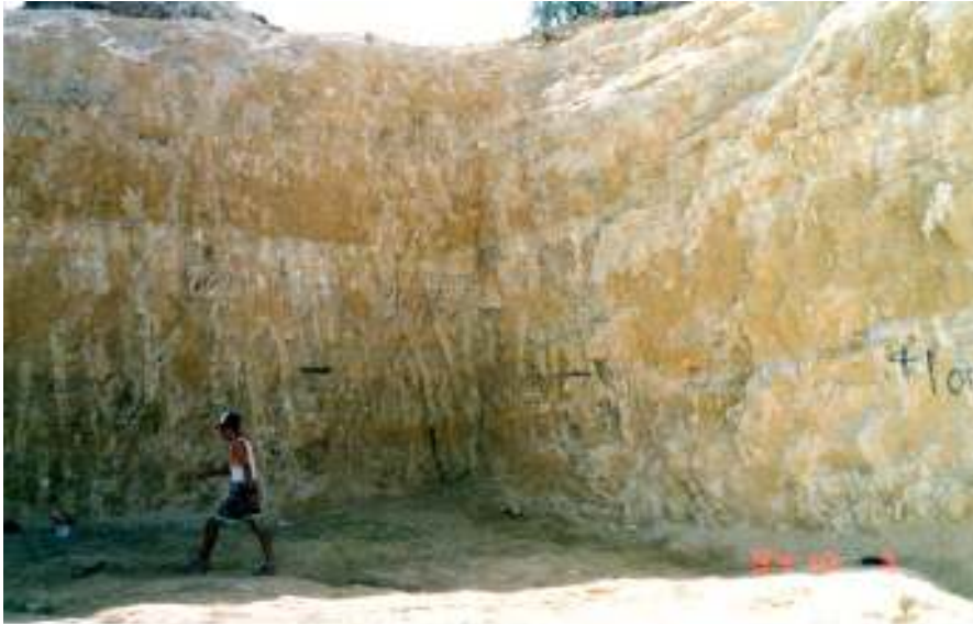
Figure 52. Foundation pit Do.
