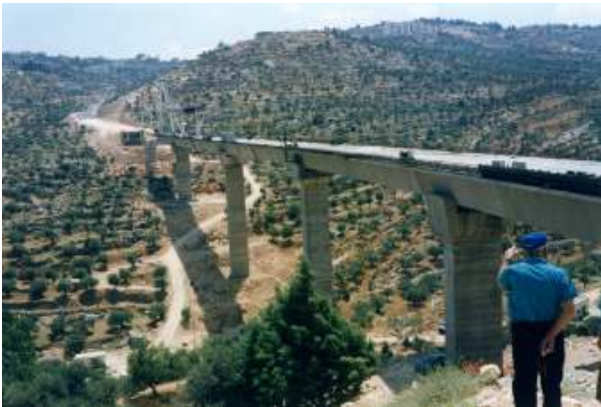
Figure 50. Gilo Viaduct during construction.
