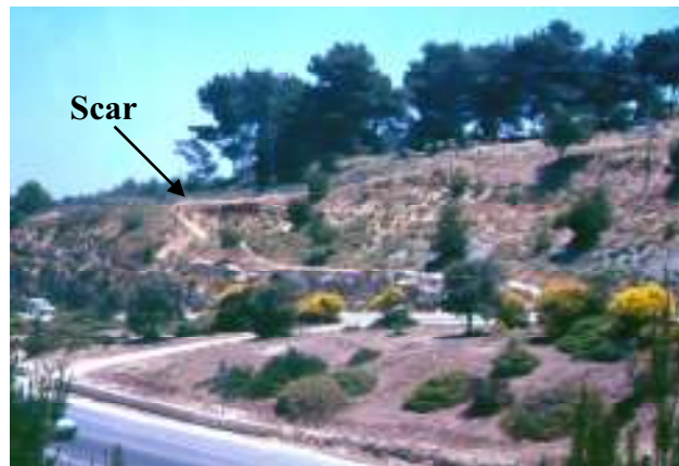
Figure 21. Circular slide and scar in the Moza marl exposure , Tel Aviv – Jerusalem highway.
