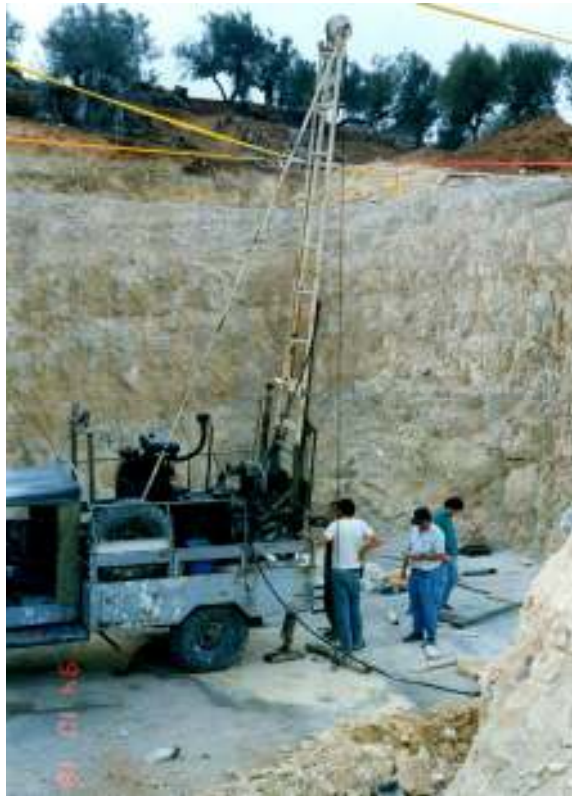
Figure 53. Foundation pit Do. Drilling exploratory and grouting holes.
