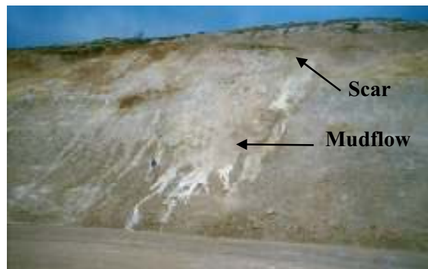
Figure 21. Circular slide and scar in the Moza marl exposure , Tel Aviv – Jerusalem highway.
