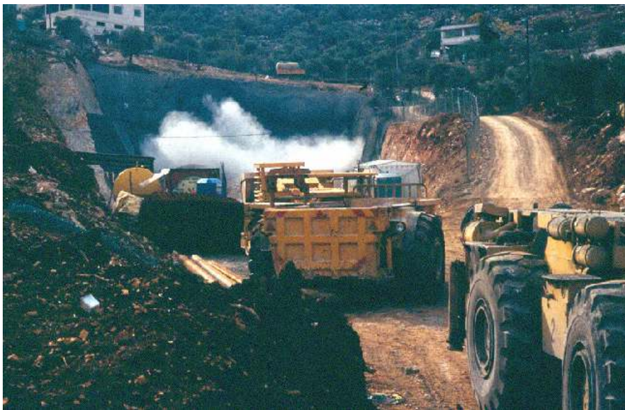
Figure 46. Gilo Long Tunnel at the start of the north portal.
