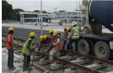
Figure 6 : Concrete pouring on KCD Staging Area
