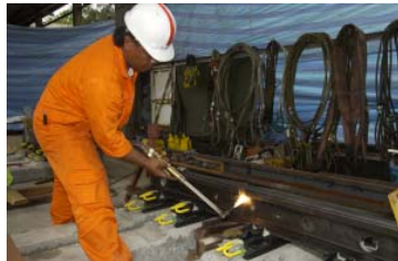
Figure 5 : Rail welding on KCD Staging Area
