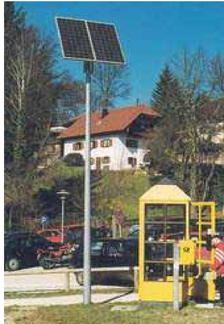
A telephone booth supplied by photovoltaics with an energy management system
