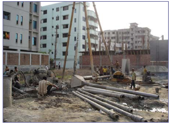
Photo - 3.13. Construction activities
