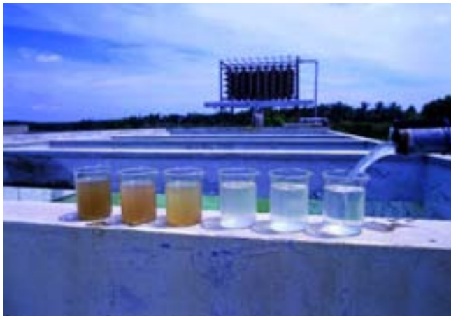
Above Water treated on site at a rubber factory, Malaysia.
