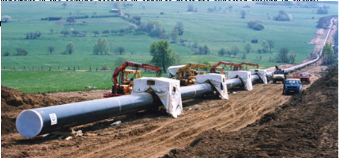
Figure 3: X80 pipeline construction in Germany. Courtesy of Europipe.
