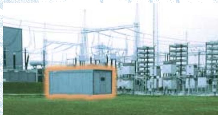
Fig. 5.4.3-5: Installation of the active AC filter, 400-kV substation Tjele (Denmark)
