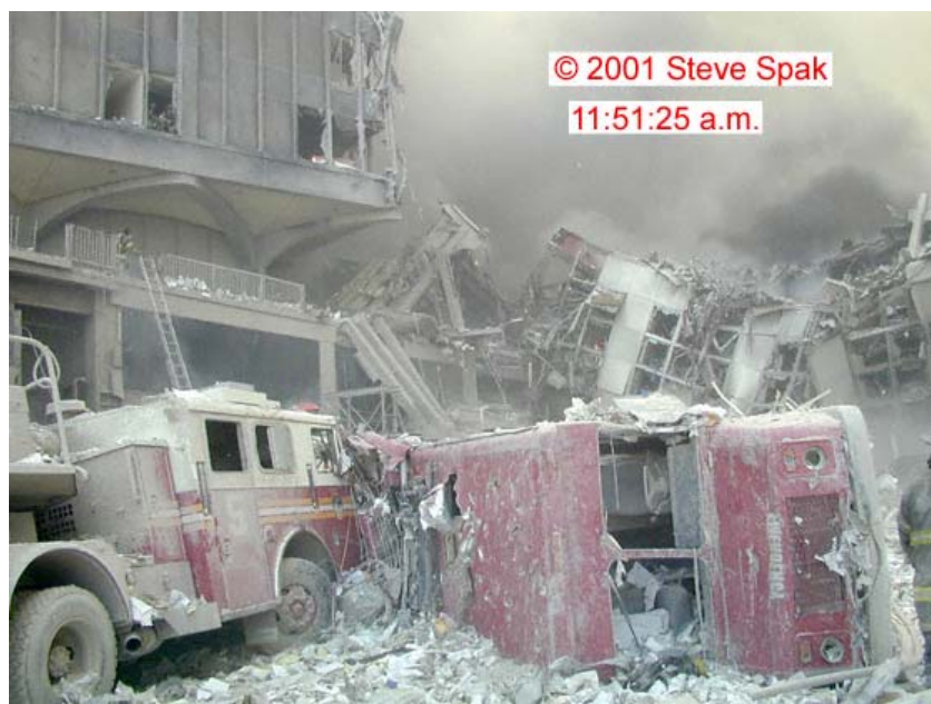
Figure 5–16. Destroyed fire apparatus following the collapse of WTC 1 and 2.
