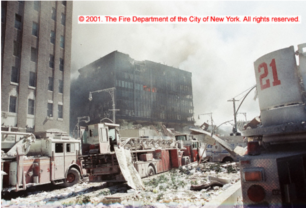
Figure 5–17. Damaged emergency apparatus at the corners of West and Vesey Street after the collapse WTC 1 and 2.
