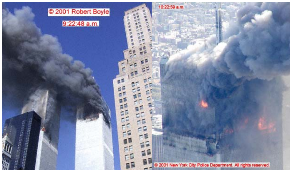
Figure 5–2. Photographs of smoke covering the roofs of the World Trade Center buildings
