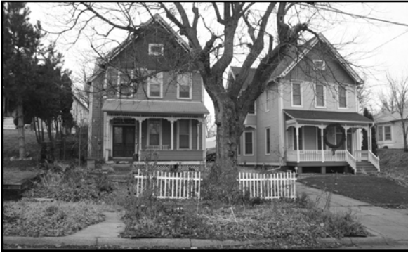
J. Grossman and the W.H. Lee Houses at 1446 and 1450 South 17 th Street as examples of Queen Anne architecture, DO09:0116-009 and DO09:0116-010
