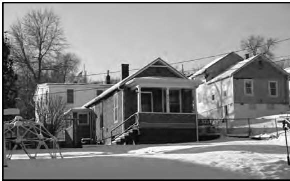
Worker cottage at 411 Woolworth Avenue, DO09:0064-066
