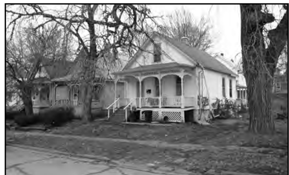
Front gable houses at 2217-2221 South 17 th Street, DO09:0114-024
