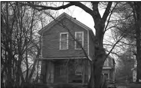
Raised-basement, front gable house at 1409 William Street, DO09:0117-072
