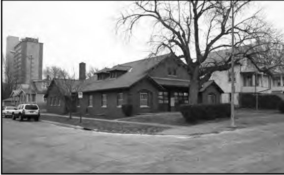
Omaha Fire Department Station at 2201 South 11 th Street, DO09:0113-050
