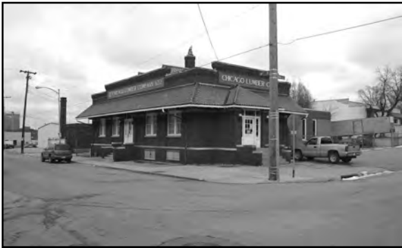
Chicago Lumber Company of Omaha Office Building at 1324 Pierce Street, DO09:0117-011
