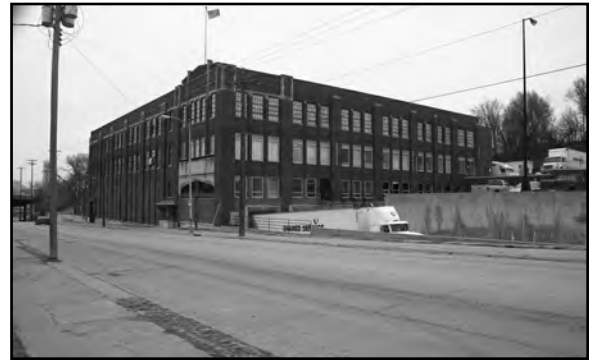
Metropolitan Utilities Distribution Warehouse and Repair Shop at 1725 South 20 th Street, DO09:0116-011
