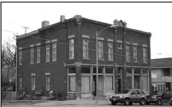
Swoboda Bakery Building at 1420 William Street, DO09:0117-012
