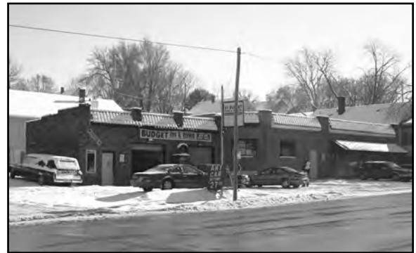
Service station at 2201 South 13 th Street, DO09:0113-036
