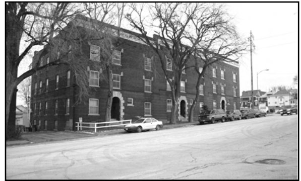
Dunsany Apartments at 1113 South 10 th Street as an example of Renaissance Revival architecture, DO09:0117-022
