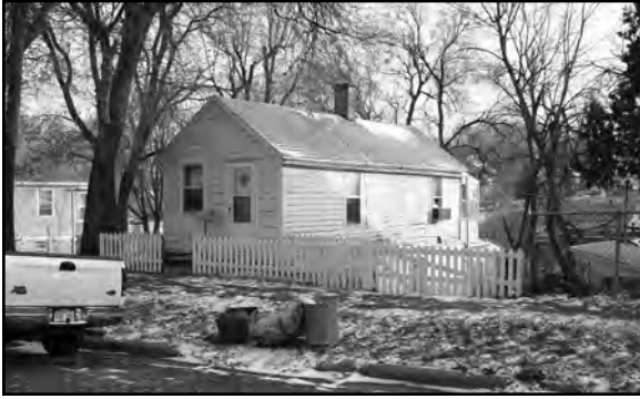
Front gable worker's cottage at 2213 South 14 th Street, DO09:0113-040
