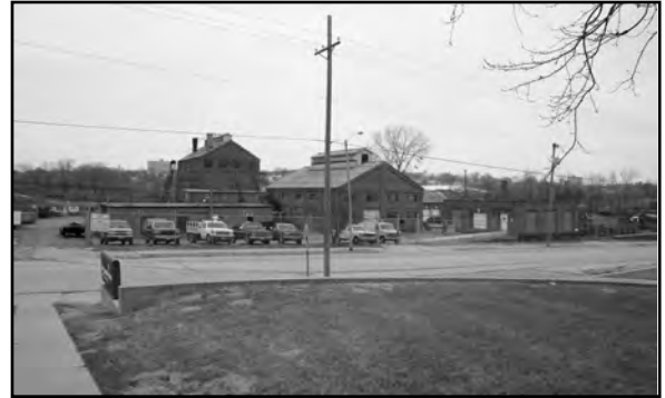
Metropolitan Utilities Distribution Gas Plant at 1824 South 20 th Street, DO09:0114-025
