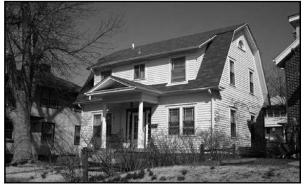
Dutch Colonial Revival house at 2418 Redick Avenue, DO09:0243-001
