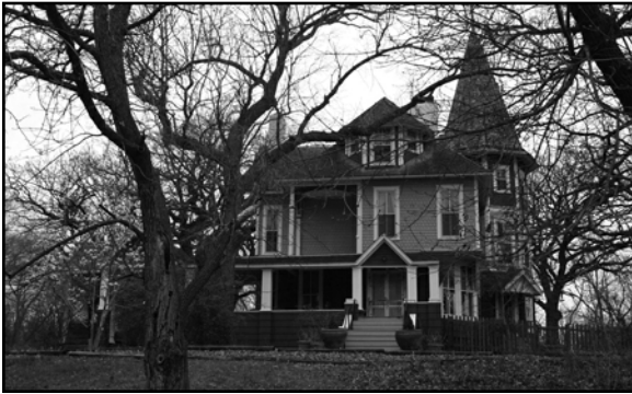
Lantry House at 3524 State Street as an example of Queen Anne architecture, DO09:0361-001
