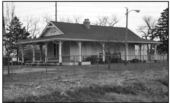
Florence Depot located between North 29th and 30th Streets, South of Dick Collins Road, (Recommended as Omaha Landmark only) DO09:0256-003
