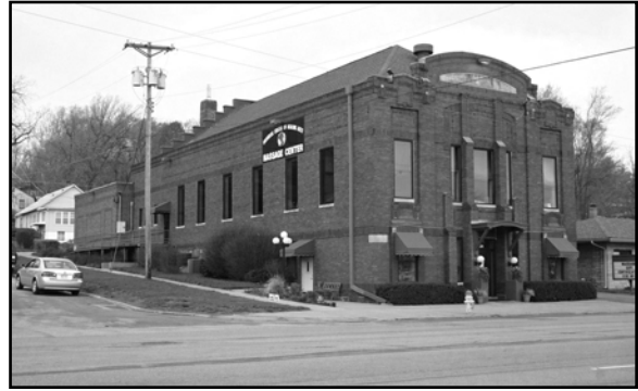
Florence Building at 8702 North 30th Street, DO09:0254-001
