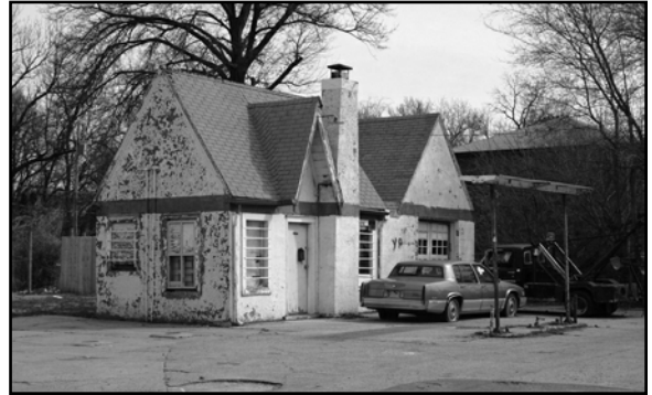
Phillips Gas Station at 5723 North 24th Street, DO09:0154-006
