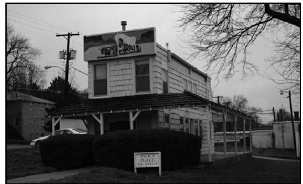
Mormon Bridge Toll House at 3010 Willit Street, DO09:0254-017
