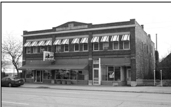
Price Building at 8607 North 30th Street, DO09:0254-004
