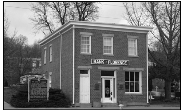
Bank of Florence located at 8502 North 30th Street, D009:0254-003 (listed in the National Register)
