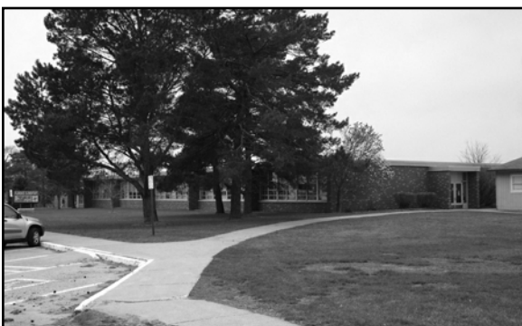
Florence Elementary School at 7902 North 36th Street, DO09:0359-007
