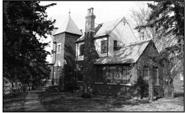
Henry B. Neef House at 2884 Iowa Street as an example of steel frame construction and Eclectic architecture, DO09:0245-001
