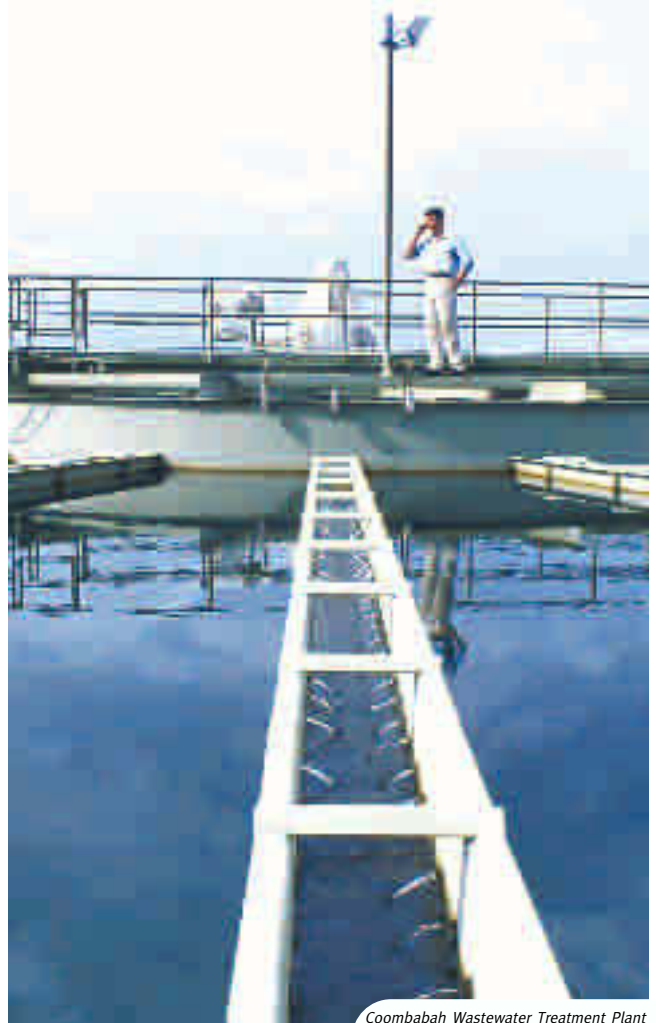
Coombabah Wastewater Treatment Plant
