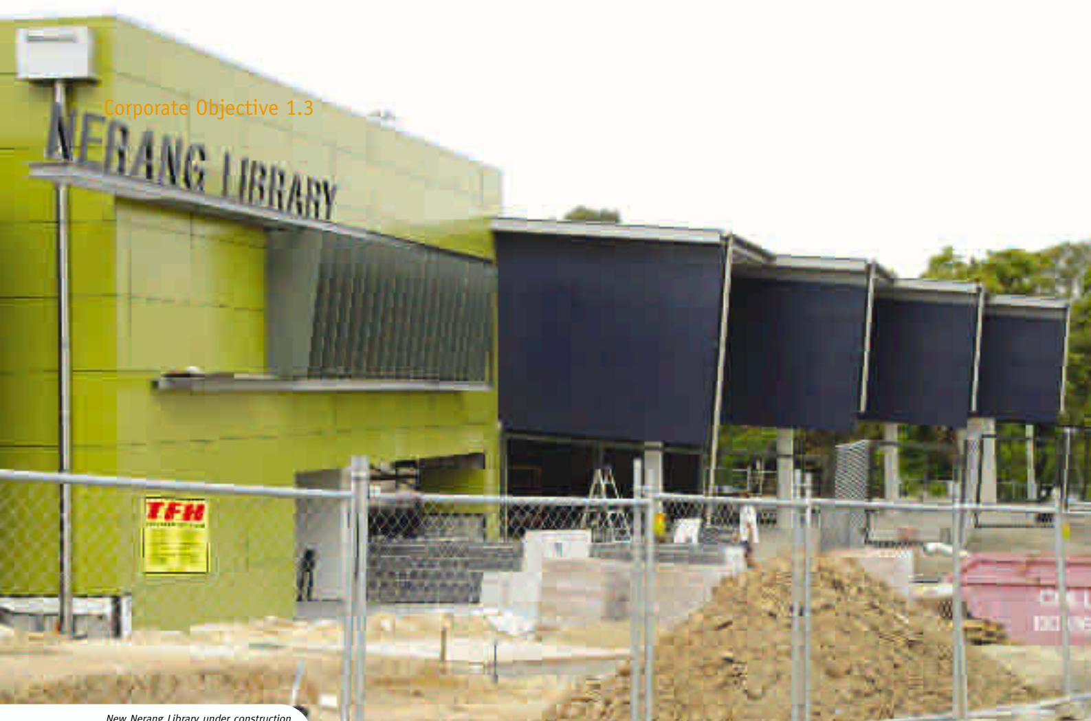
New Nerang Library under construction
