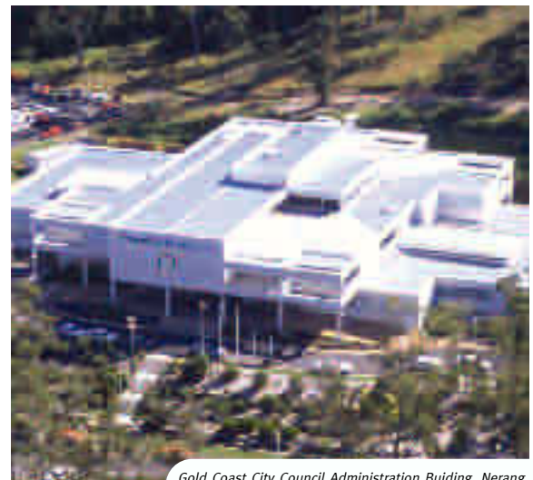
Gold Coast City Council Administration Building, Nerang
