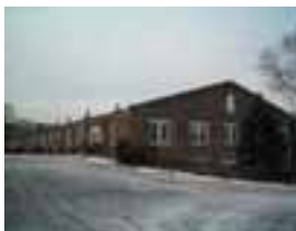
Building 110 Office building Location: Arsenal District Details: Romanesque Revival style, two-story building, total floor area of 47,934 square feet
