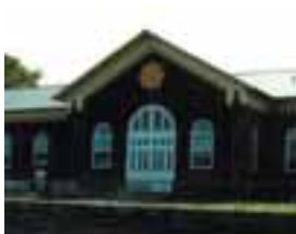
Building 140 Office Building Location: Arsenal District Details: Romanesque Revival structure, one-story building, total floor area of 7,950 square feet; with 1,000 square foot NPS easement
