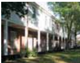
Building 25 Office building Location: Arsenal District Details: Utilitarian structure, two-stories in the front and three-stories in the rear, total floor area of 13,540 square feet
