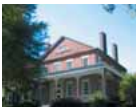
Building 135 Commander's House Office/Two-family house Location: Arsenal District Details: Greek Revival/Utilitarian, wings with two, two-and-a-half, and three-, stories, total floor area of 14,865 square feet
