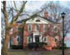
Building 2 The Governors House Location: Nolan Park Details: Georgian structure, two-family house, two-stories, 5,983 square feet total floor area
