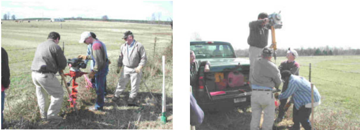
Figure 8-10. Setting deep-driven benchmarks (Memphis District & 3001, Inc.)
