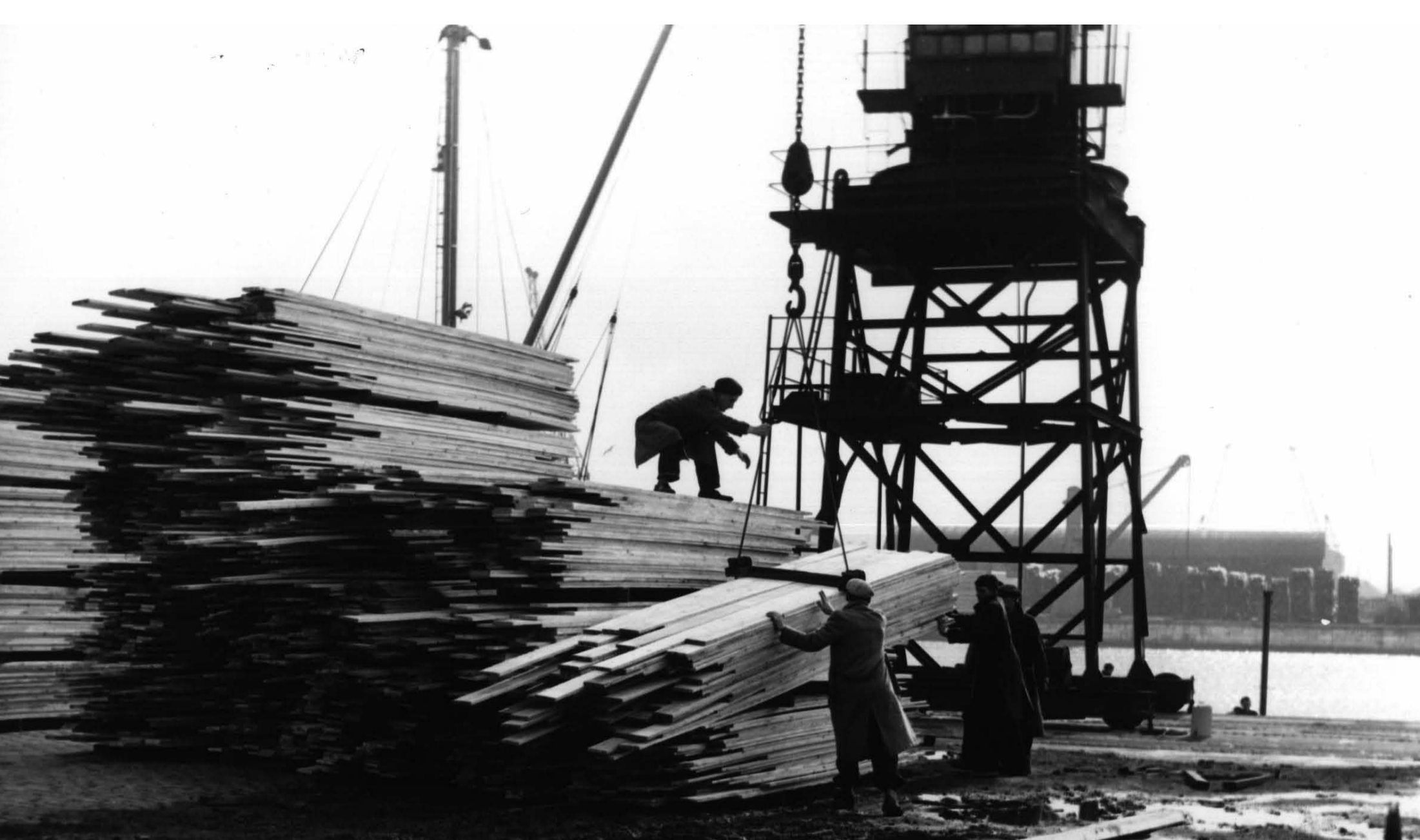
Unloading Timber at Millbay using Pearce's 'Plymouth Gear' Associated British Ports Collection, Southampton City Heritage
