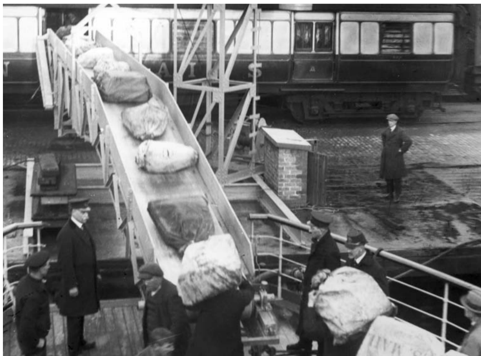
The newly installed electric conveyor for unloading mail sacks, 1927 Plymouth Library Services
