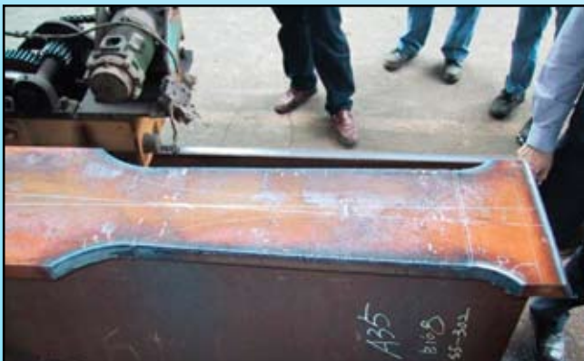
Figure 12: Tapered flange trimming at selected link beams creates a 'dogbone' condition to improve ductility by locating beam yield zones away from welded joints.
