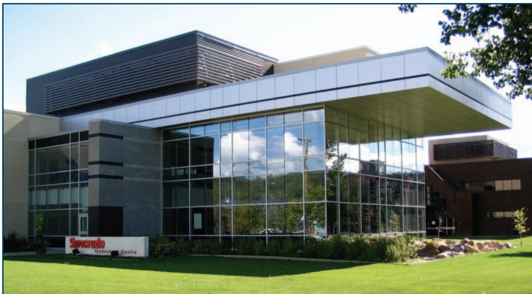
The Syncrude Technology Centre at Keyano College, Fort McMurray
