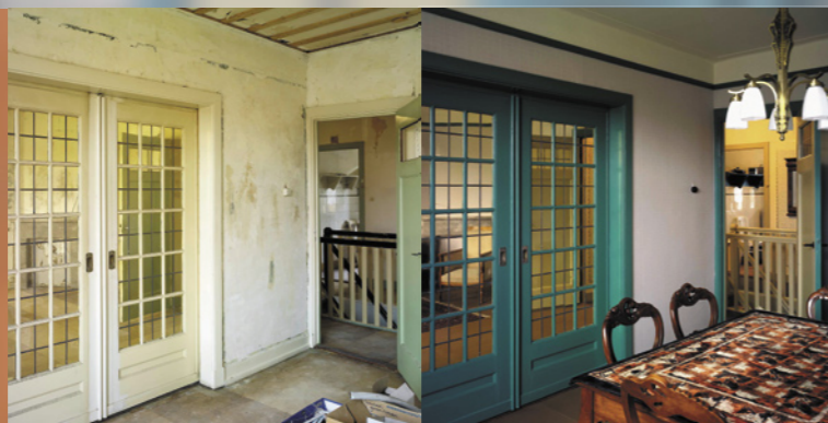
The living room of the former residence of the Frank family before and after the restoration.
