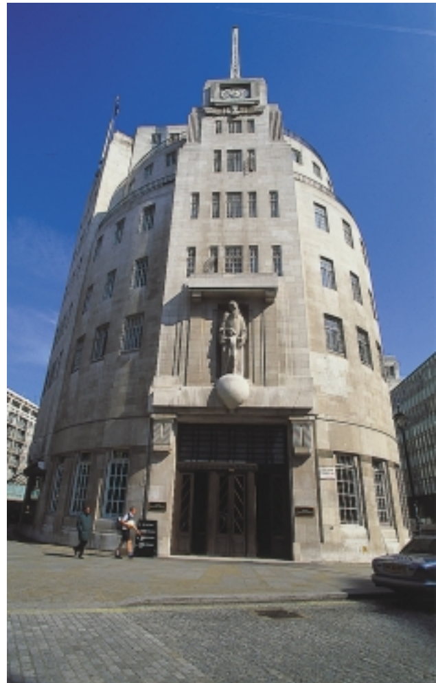
Broadcasting House, Portland Place, London W1: on part of the site once stood a pub called "The Devonshire Arms", the first property to be compulsorily registered on 9 January 1899, (Title Number 20001). (Photo: Ian Stone)
