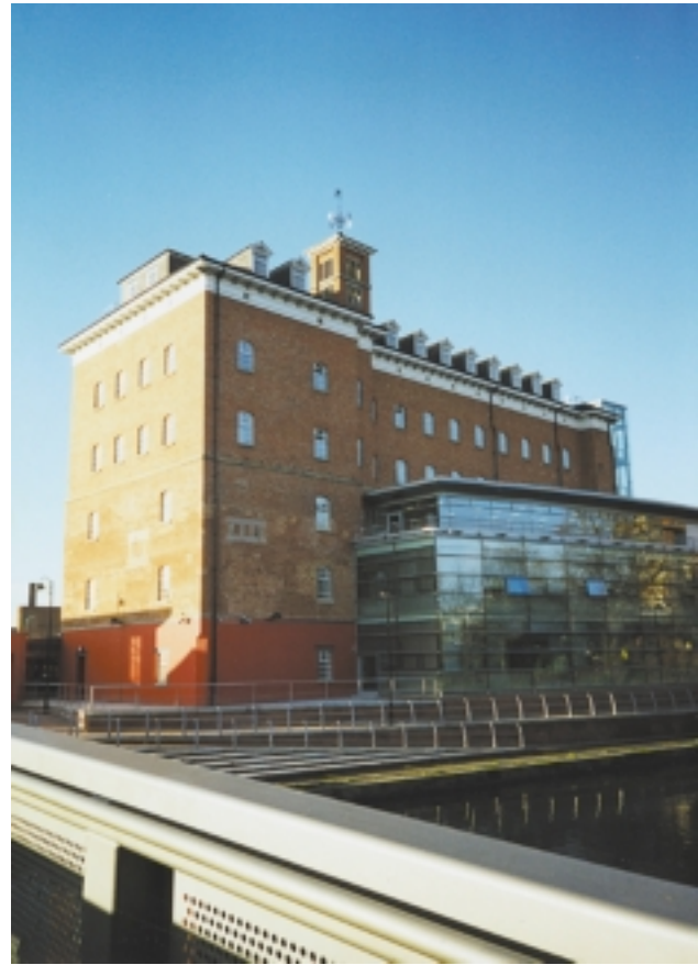
Leicester District Land Registry, (formerly a factory, it is one of the Land Registry's newest offices, but its oldest building).
