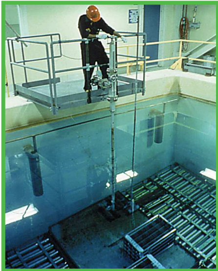
Used fuel is stored for at least 10 years under water in fuel bays at Darlington Nuclear. The water keeps the fuel bundles cool and provides an effective radiation shield.
