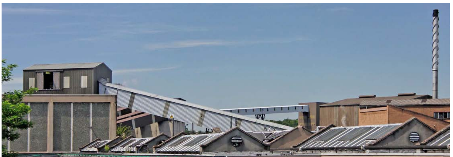
Drift mine - conveyors bring the coal to the surface
