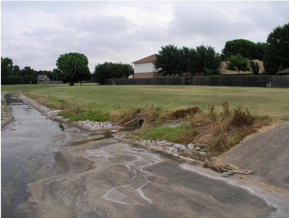
Valley View Creek looking upstream from Pleasantview Drive before recommended improvement.
