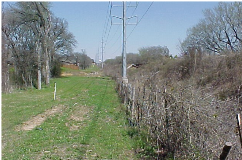
View of the TXU and railroad corridor along which the Cottonbelt Trail is to be constructed.
