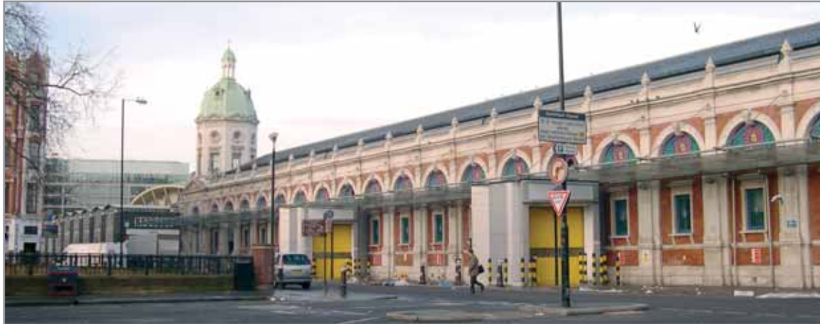
View looking west along West Smithfield towards Smithfield Market
