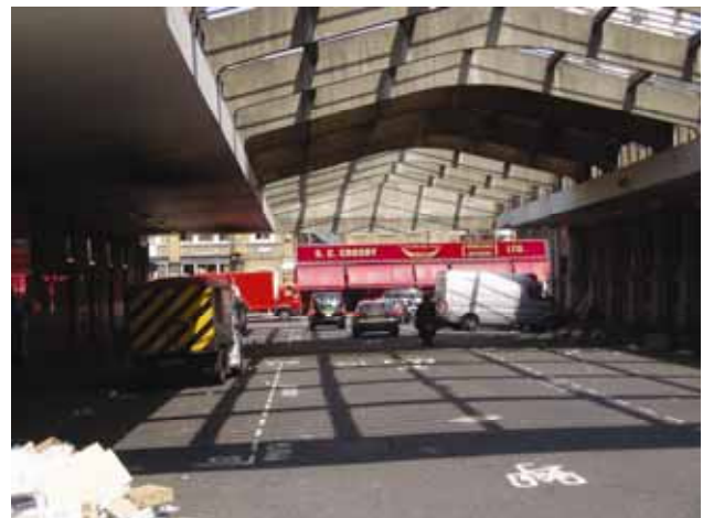
View along East Poultry Avenue towards 65/65a/65b Charterhouse Street
