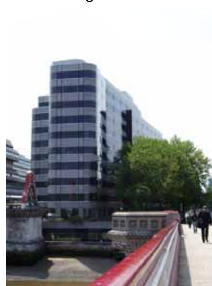
View of Ludgate House
