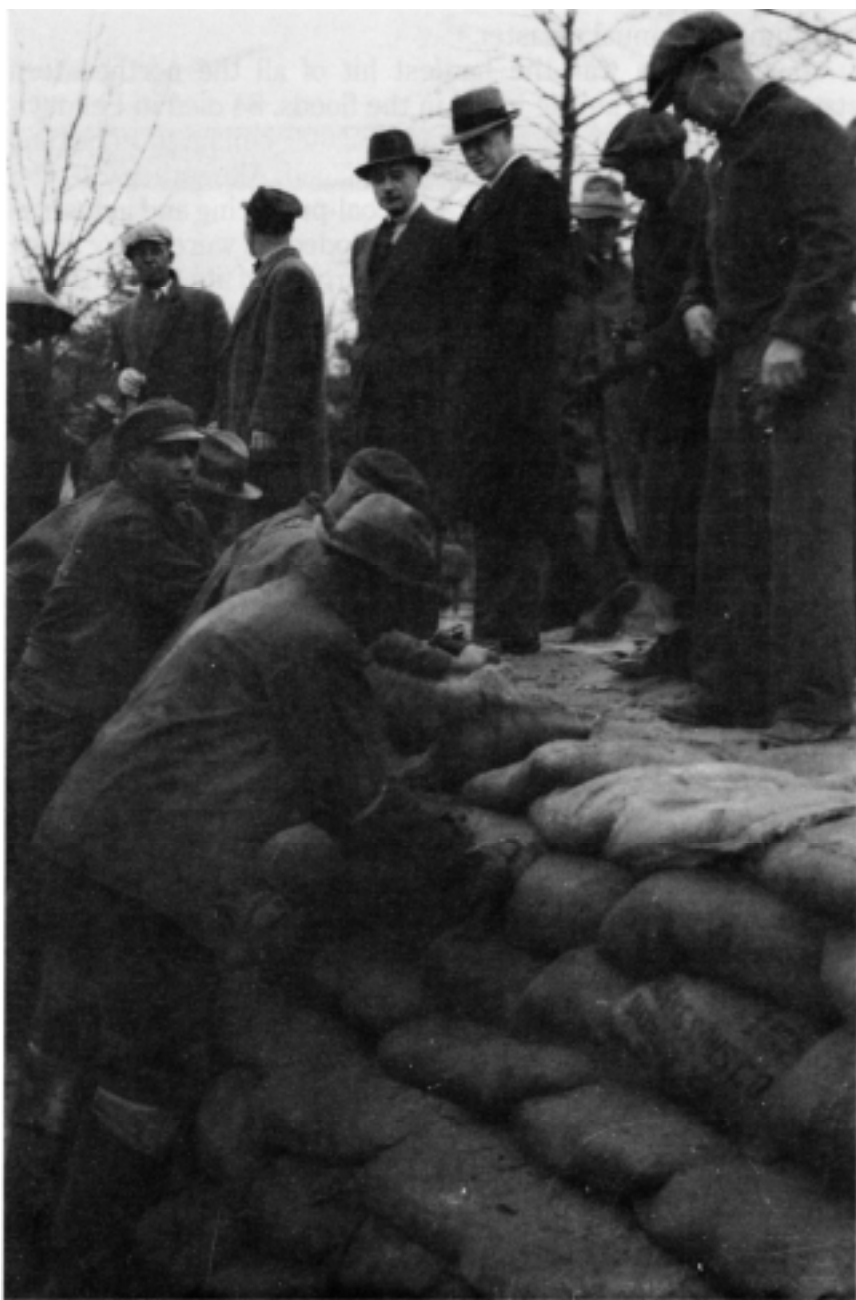
Engineer Lieutenant Colonel Francis C. Hawington (above, left center) with the Works Progress Administration, and Harry L. Hopkins (right center), Administrator of the WPA, watching workmen erect an emergency levee in rear of Munitions Building, Washington, DC, March 1936.
