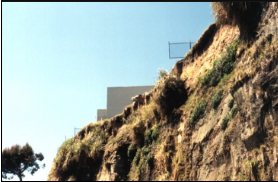
Fig. 80: Retreating cliff due to undercutting by wave erosion at Capitola Beach.
