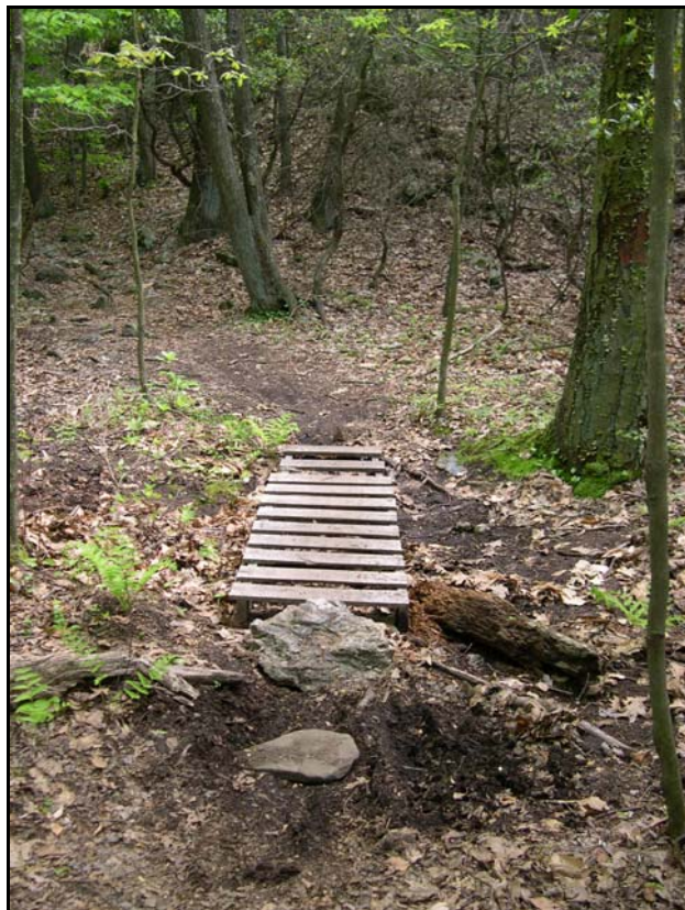
Figure 44. ORV tracks skirt a footbridge, creating ruts in a streambed at Reservoir Loop.
