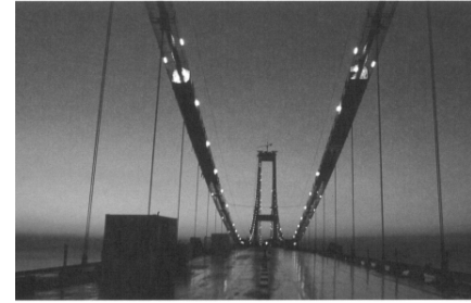
The new Storebælt bridge, which connects Funen and Zealand.
