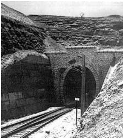
Arhivski snimak ulaza u tunel Dujmovača (Split predgrade)
