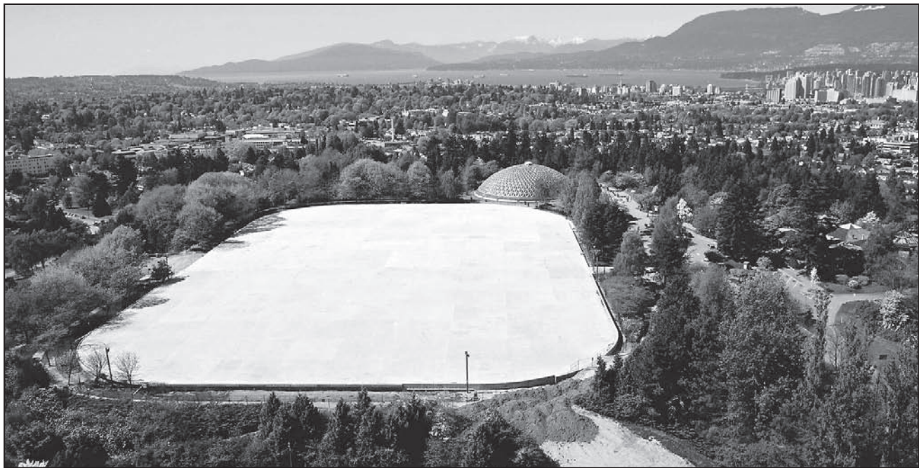
Participation from the public helped the GVRD to complete the reconstruction by February 2004. This is the area the VPB will redevelop. See the current plans of the cover of this fact sheet.
