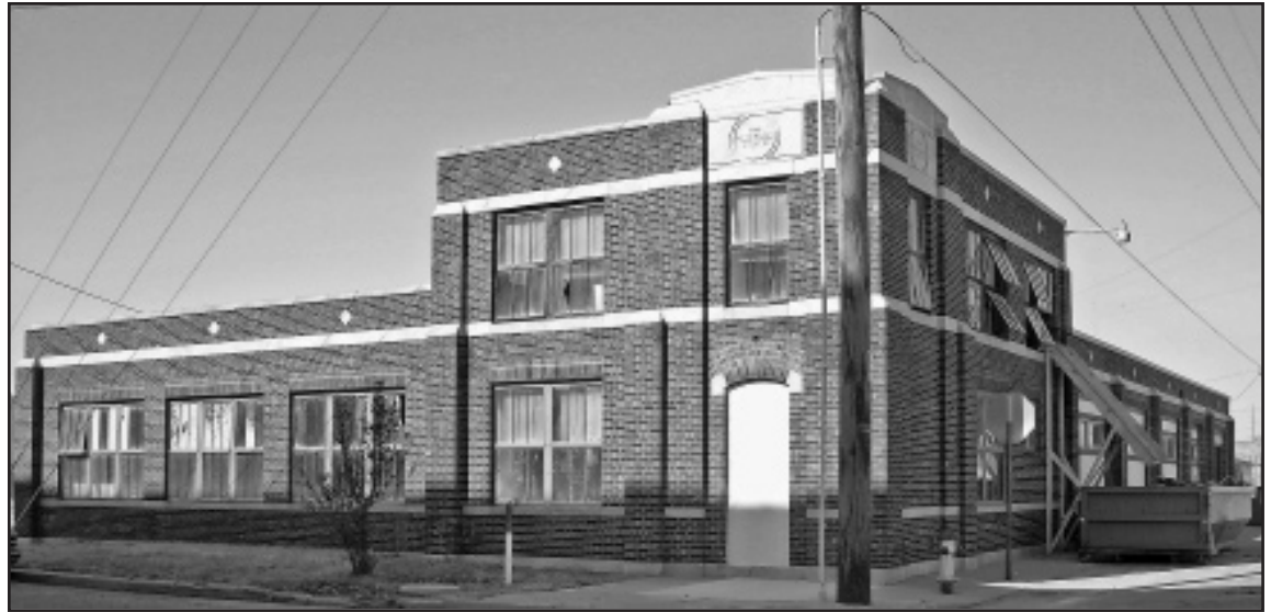
Built in 1929, Wichita’s Keep Klean Building is an example of fireproof industrial construction.
