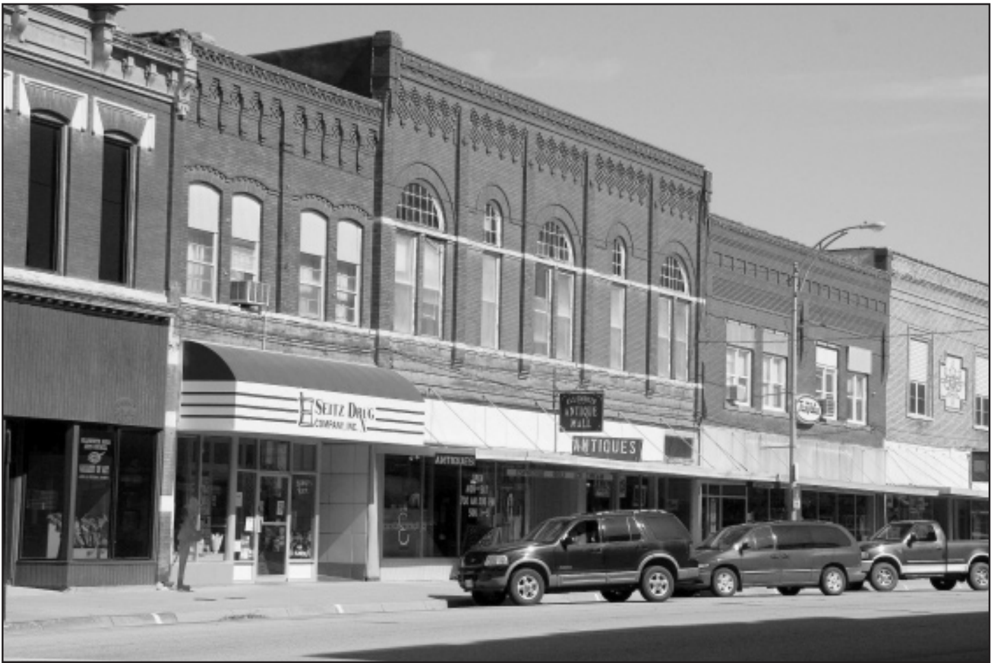
The Ellsworth Downtown Historic District is comprised of eighty-seven structures dating from the town's early cowtown days through the mid-twentieth century.
