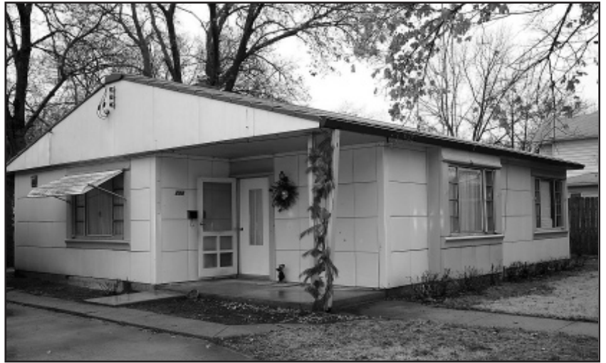
Lustron Homes, like the Berger House in Abilene, are easily identified by their porcelain enamel-coated steele panels.
