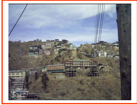
New construction underway ....
