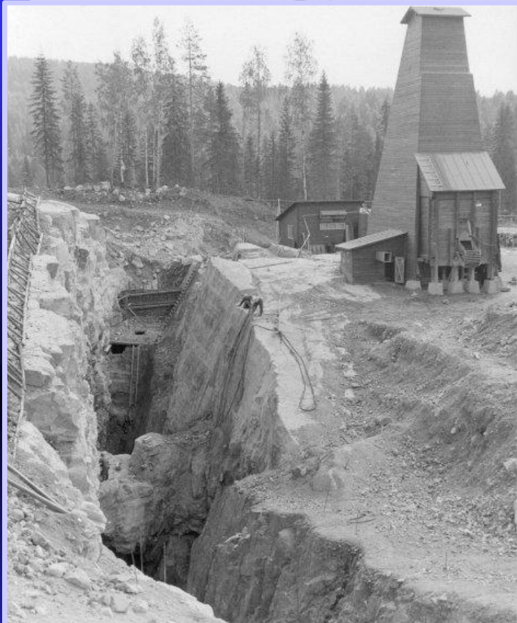
Paukkajanvaara mine in summer 1961, just before closing the mine. The right wall of the pit is the contact between quartzite and dolerite. Mineralised, sheared dolerite still left in the central part of the pit and in the front area of the view. Photo courtesy Matti Tyni.
