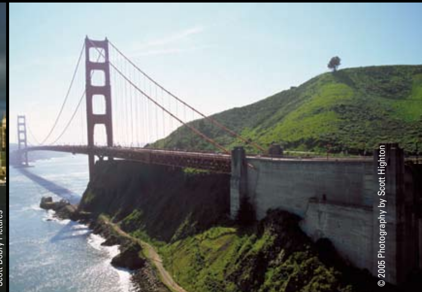
Golden Gate Bridge Phase IIIA Seismic Retrofit
