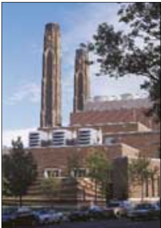
1 Sterling Power Plant at the Medical Center 2 Central Power Plant
