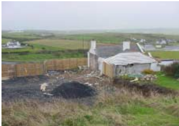
And this shows a listed property at the entrance to the site, which has been partly demolished by its owner to make way for a Arts Crafts and Cultural Centre, which we feel would seriously compromise the context of the World Heritage Site.
