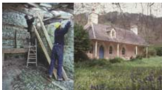
Carpenter and assistant measuring a length of replacement timber in the roof of cattle sheds at Llanerchaeron Farm. The wood will be cut with an adze beforehand and pegged with wooden pegs. The charming C18th Estate Office at Llanerchaeron, set in a field of bluebells. The rough stonework of the cottage is painted pink and white and the windows and doorframe are arched.
