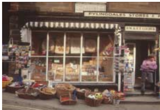
The exterior of the General Store, Bay Town, Robin Hood's Bay
