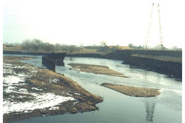
Figure 7: The Mersey at Urmston in March 1983 (top) and in early 1986 (bottom) showing how shift to the channel caused the iron piling put into to protect the pylon on one bank ended up on the other side of the channel. (The piling was removed around 1990).
