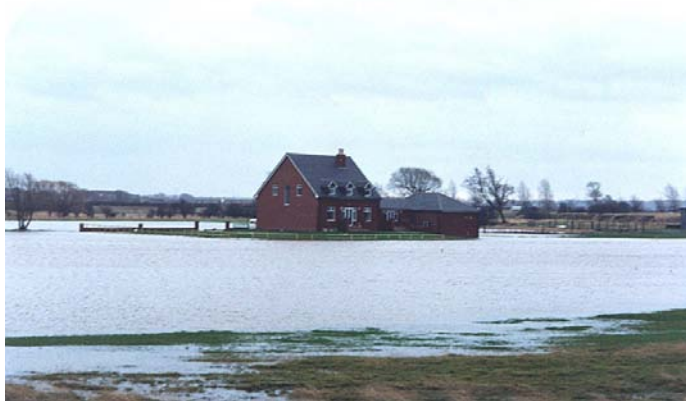
Figure 6: Floodwaters around Willow Farm in the Mersey floodplain, 27 December 1991.
