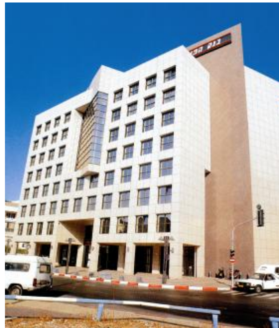
Fig 2.1.6 Existing Hapoalim Bank Headquarters in T.A.Y's CBD
