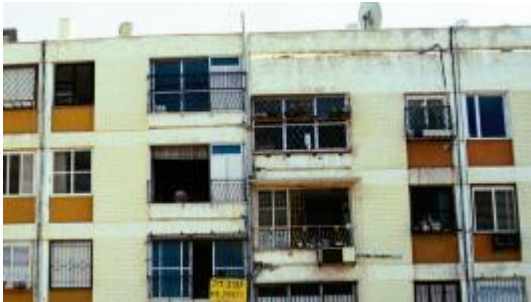
Fig 2.3.3 Example of an old residential area in South T.A.Y
