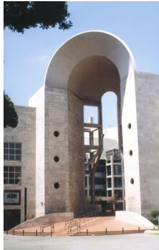
Fig 2.1.11 The Centre for the Performing Arts
