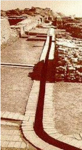
A brick-lined drain. Mohenjodaro
