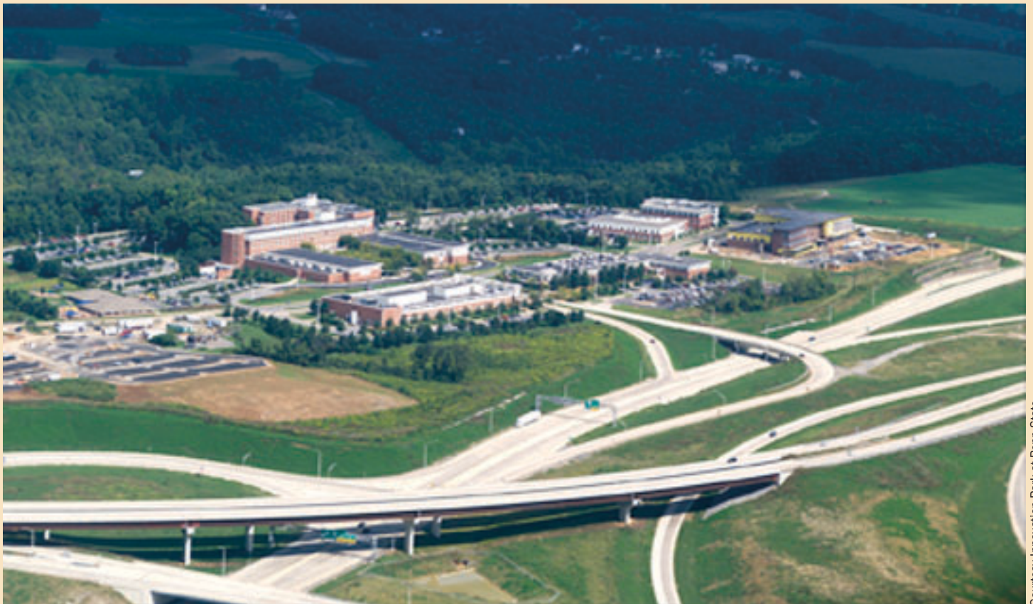
Aerial view of Innovation Park at Penn State
