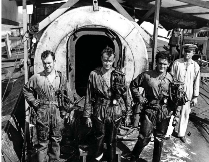
Divers standing in front of a decompression chamber, while they were working to salvage ships sunk in the 7 December 1941 Japanese air raid on Pearl Harbor.
