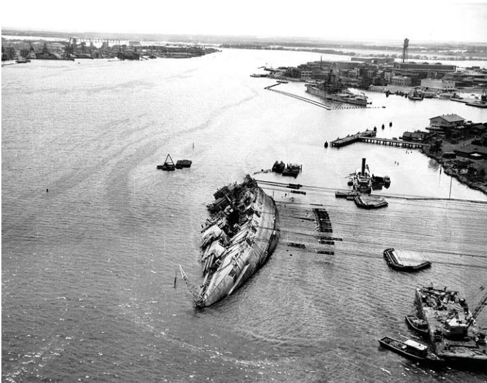
USS OKLAHOMA (BB 37) Ship righted to about 30 degrees, on 29 March 1943, while she was under salvage at Pearl Harbor. She had capsized and sunk after receiving massive torpedo damage during the 7 December 1941 Japanese air raid. Ford Island is at right and the Pearl Harbor Navy Yard is in the left distance.
