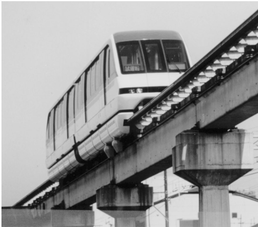
HSST-100L vehicle on elevated test track in Nagoya City
